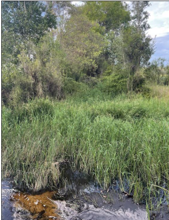
Photo 7 – Existing main drain which bisects the subject site generally in a north south direction
